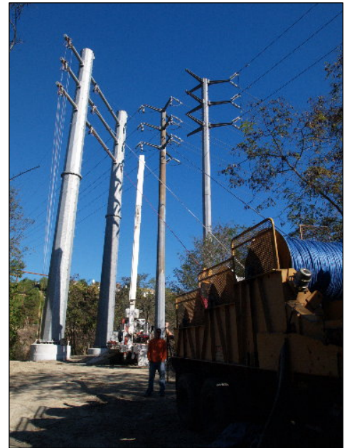
The pulling phase of a wire-stringing operation. Note the reel of conductor on the right side of the photo.
