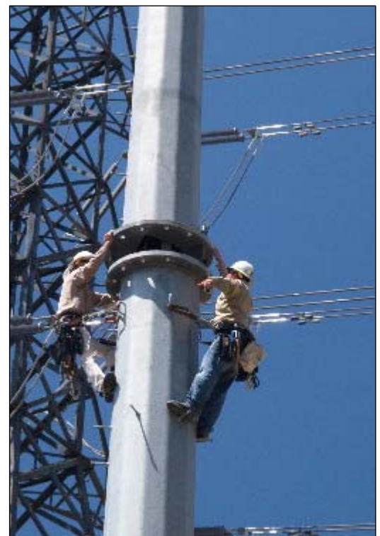
Crews joining the sections of a TSP.
