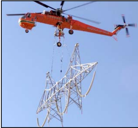
An Erickson Air-Crane carries the top section of a LST for installation.
