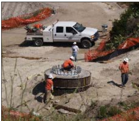
Foundation construction for a TSP.
