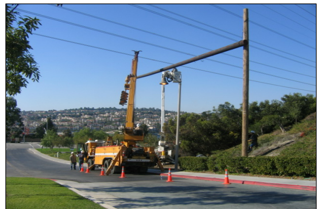
A guard structure being erected at a street crossing.
