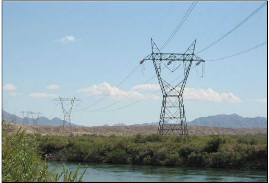
A transmission line composed of single-circuit lattice steel towers (LST). Note the three sets of bundled conductors (wires) which combine to make one circuit. The two triangular structures at the top of each tower support the ground wires (two per tower in this photo).
